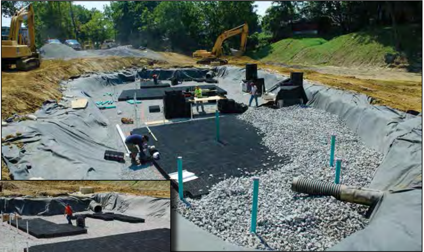
Installation of impervious liner, matrix boxes and gravel.
