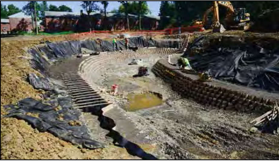
Above: Construction of forebay. Below: Installation of Geo Web liner in forebay.
