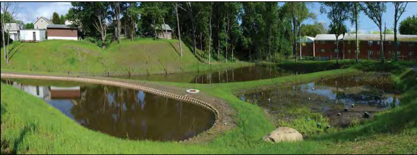
Wappingers Stormwater System at work.
