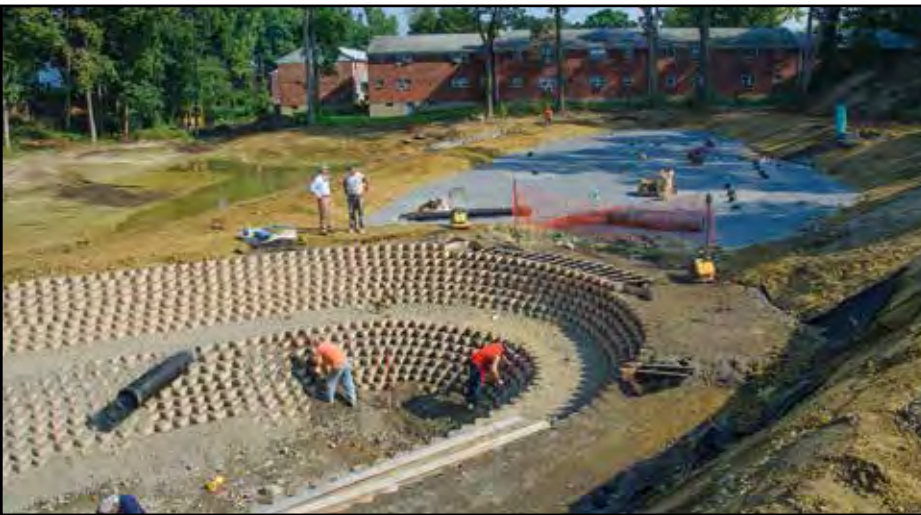
Above: Construction of forebay. Below: Installation of Geo Web liner in forebay.
